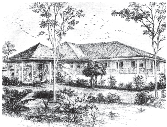
Fig. 12.23 A bungalow in Bombay, nineteenth century
