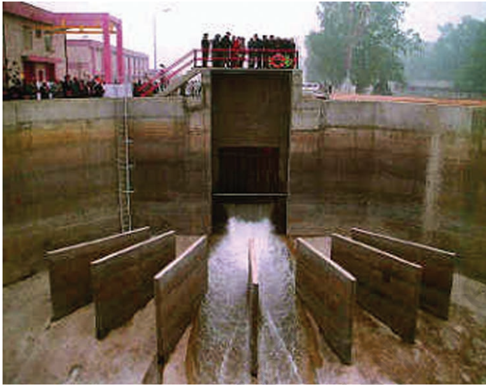
Fig. 18.10 : Water treatment plant
