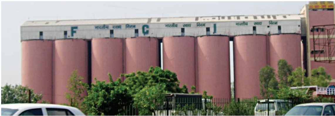
Fig. 1.10 (a) : Silos for storage of grains
