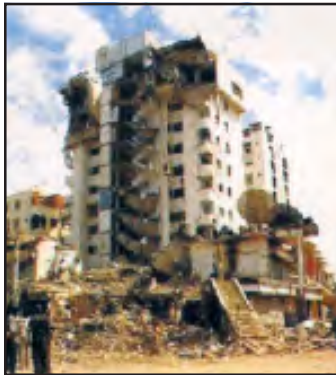
Fig. 3.3a: Destruction caused by an Earthquake in Gujarat
