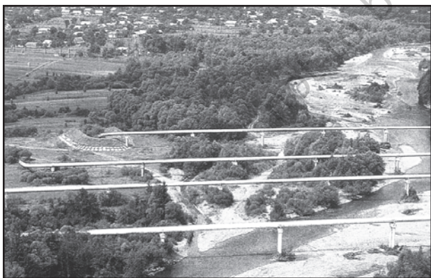
Fig. 8.17: Pipelines transporting natural gas in Ukraine
